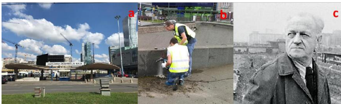
Figure 3.5. Śródmieście WKD Station Pavilion. (a) General view, (b) sampling on the monument, and (c) Arseniusz Romanowicz.
