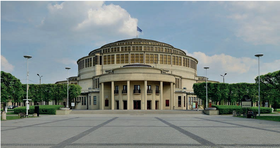
The Centennial Hall: one of the most iconic concrete buildings from the 20th century
